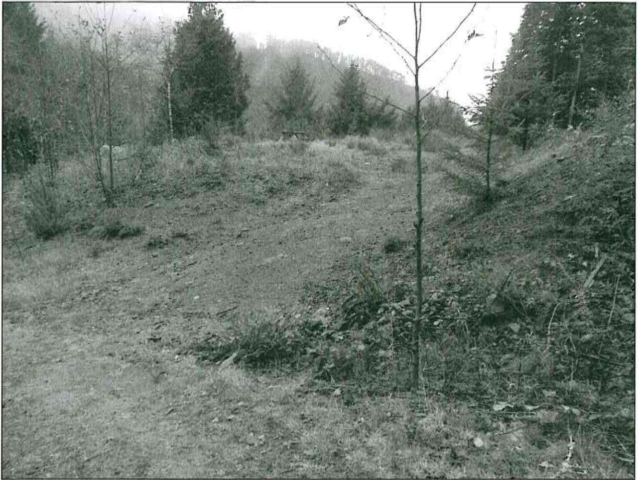
Figure 5: View of driveway ramp on east side of TL 3000, looking southwesterly. Blocks of basaltic rubble are up to 2 ft across in the exposed ground and may be larger in the shallow subsurface.
